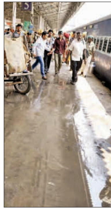
FACELIFT NEEDED: Railway station has several areas that need attention
